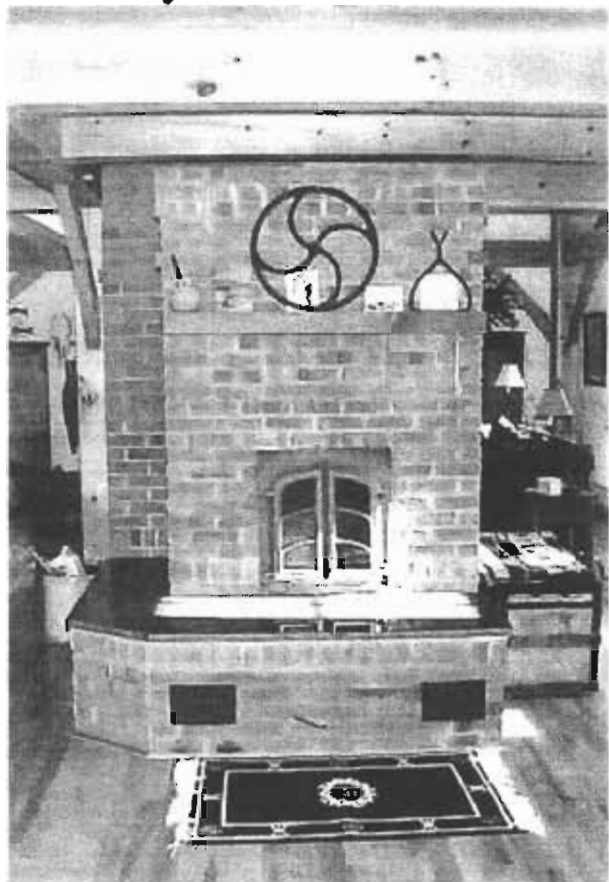
C-MAST: HK 22 w. heated bench. Plattsburgh, NY. Mason: Dan Pike .
