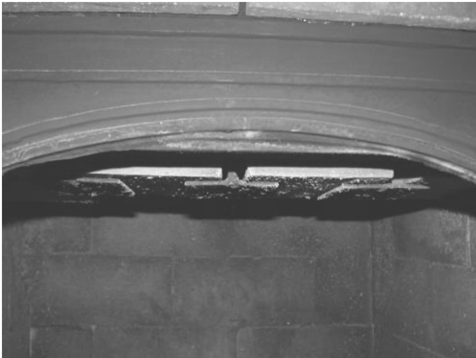
Figure 4. Location of heat shield bricks relative to door.
