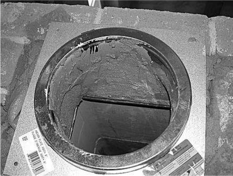
The photo above shows a castable refractory transition parged into place, before cleanup and sponging smooth.
