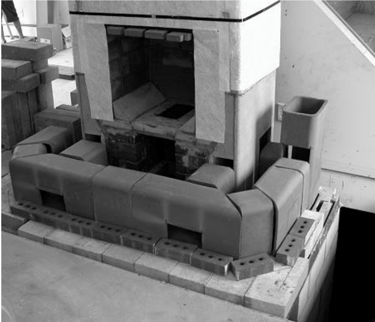
Figure 3. Dry Heated Bench layout and chimney connection
