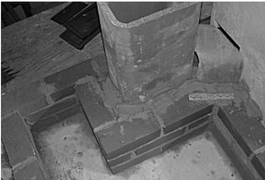
Figure 5. Mortar slush around flue liners.
