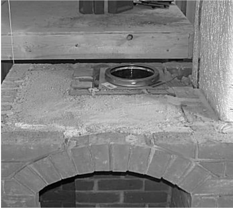
Figure 6. Metal chimney connection
