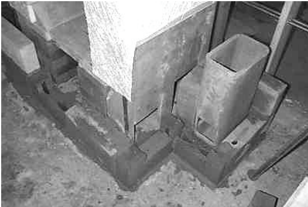
Figure 1. Typical Chimney Connection
