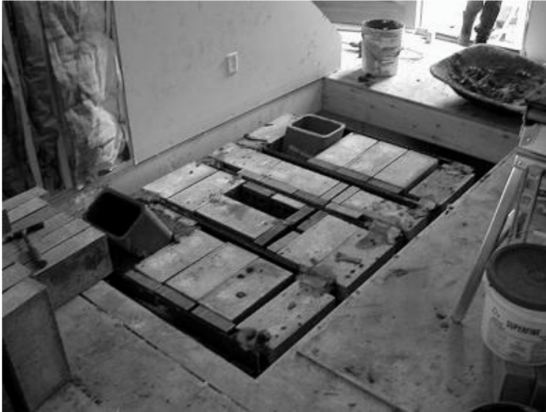
Figure 2. Chimneys coming up through foundation.
