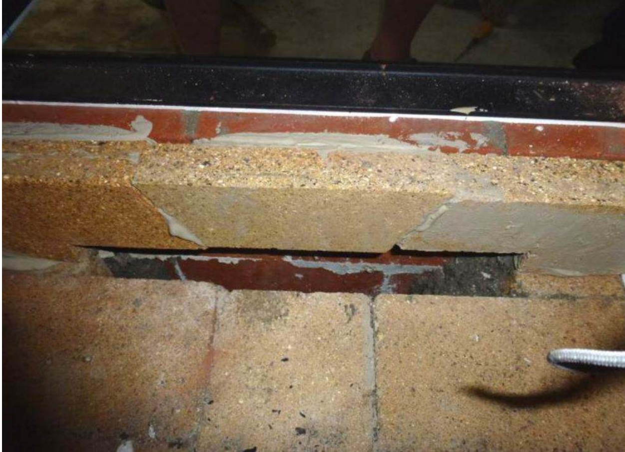
View of bottom of door, from inside the firebox, showing air slot created with firebrick splits
