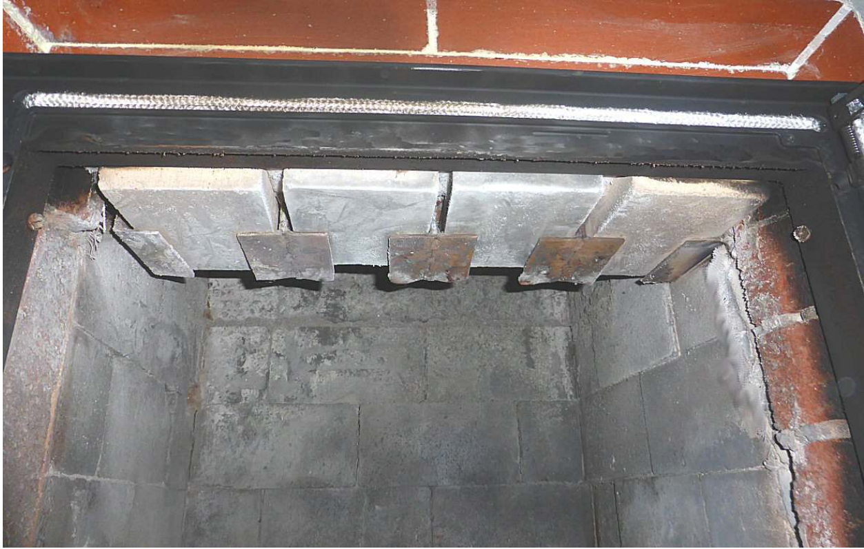
Figure 3. Location of heat shield bricks relative to door.
