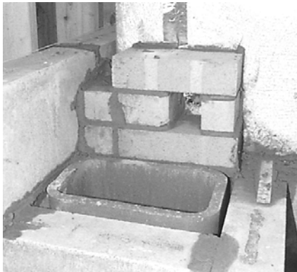
Gas slot detail
